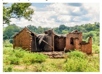
(NB this is an unusually large house but the damage caused by the rain is obvious. For most
