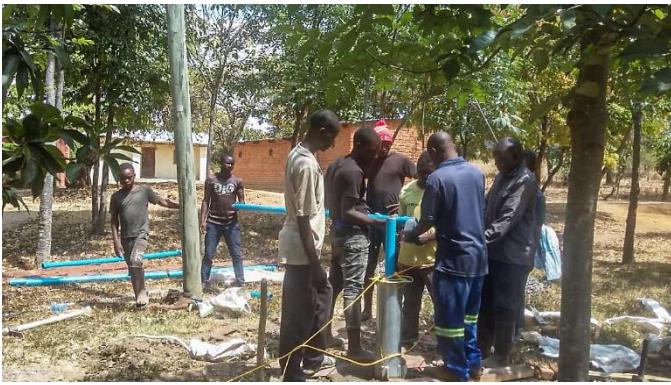
Installing the new manual water pump at the Village of Light
